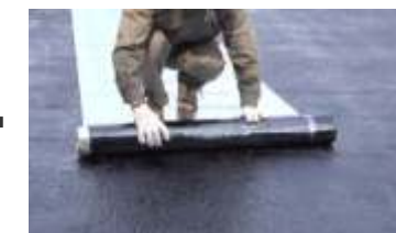
Paste Self-adhesive Waterproofing Membrane
