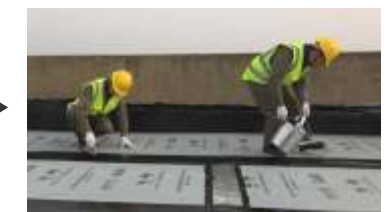
Grouting Treatment (For WICI MAC-type)
