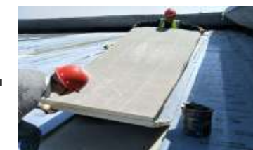
Pre-pave WICI Panels, Positioning and Snapping the Line
