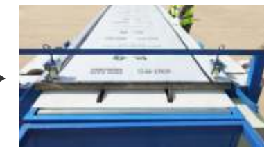
Cut WICI Panels
